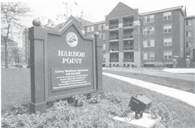
Fig. 8. The failed Columbia Point public housing project was converted to mixed income “luxury apartments” at Harbor Point.
